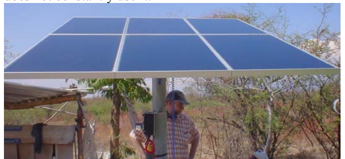
Fig. 6: El Laurel PV Array under test by NMSU and UNAM.
