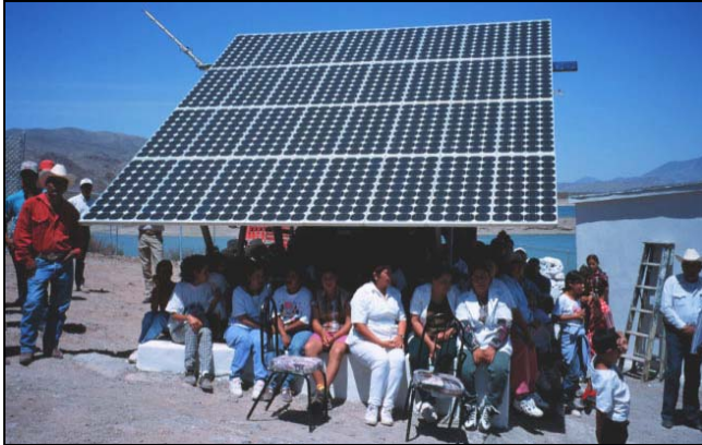
Figure 3. World's first PV ice-maker developed by SunWize for the fishermen of Chihuahua (1999).
