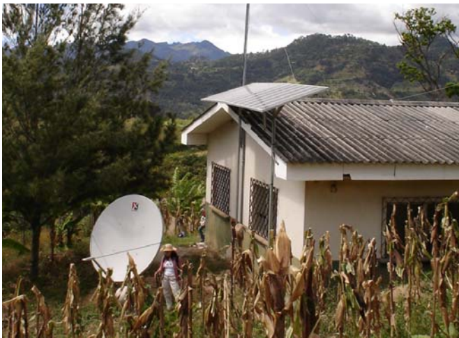
Fig. 5. San Manuel Colohete 700 Wp PV array and satellite communication system in Lempira Department.
