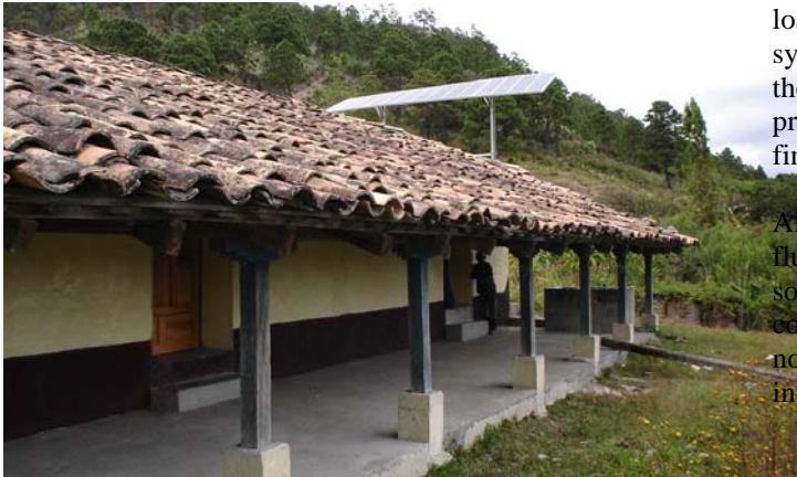
Fig. 7. San Francisco telecenter with 700 W PV array.
