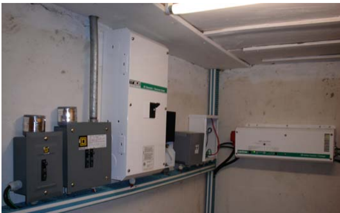
Fig. 8. San Francisco telecenter components and 20W fluorescent light. Note the Trace 1500 W DR 1512 series sine wave inverter on the far wall.
